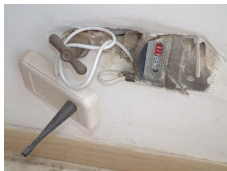
Figure 5: Zigbee-based AMR latched onto the consumer water meter
